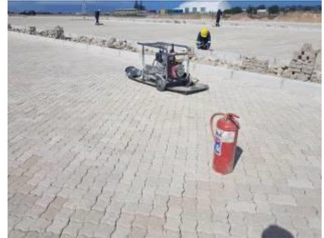
Image 9: Generator, drip tray and fire extinguisher on site.
