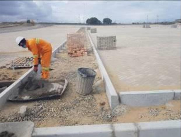
Image 19: Mixing of cement on an impermeable surface with a waste receptical close by.
