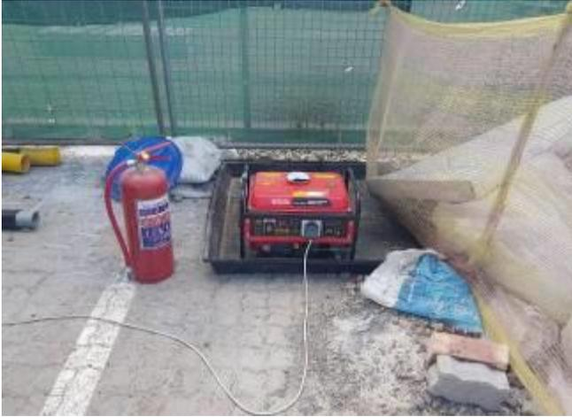
Image 1: Drip tray and fire extinguisher in place.
